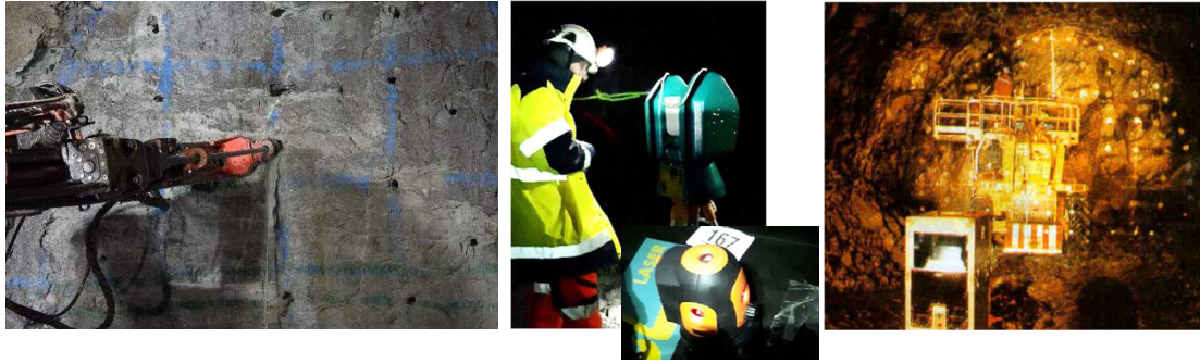
Figure 5: grid paint of face (left) --- laser system projecting hole mark according to drilling pattern (center) --- drill plan projected directly on the face with a digital projector (right)
